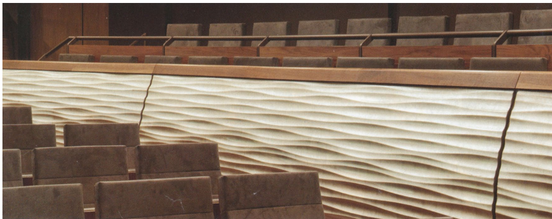
Figure 40. Patterned Balcony Fronts at Winspear Opera House. Photo from Architectural Record (2010, February).
