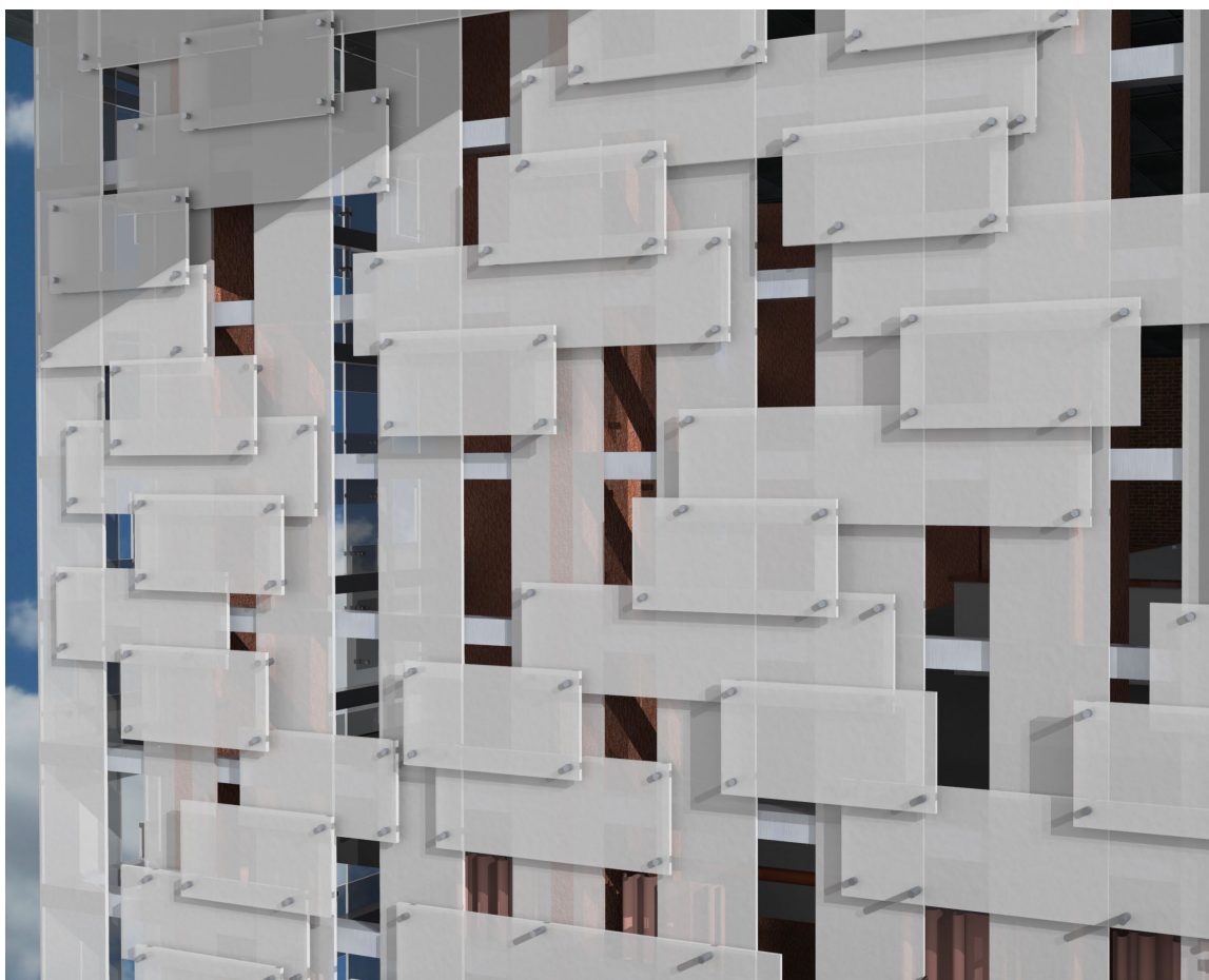
Figure 68. Detail View of Frosted Glass Panel Exterior Skin. Image by author.
